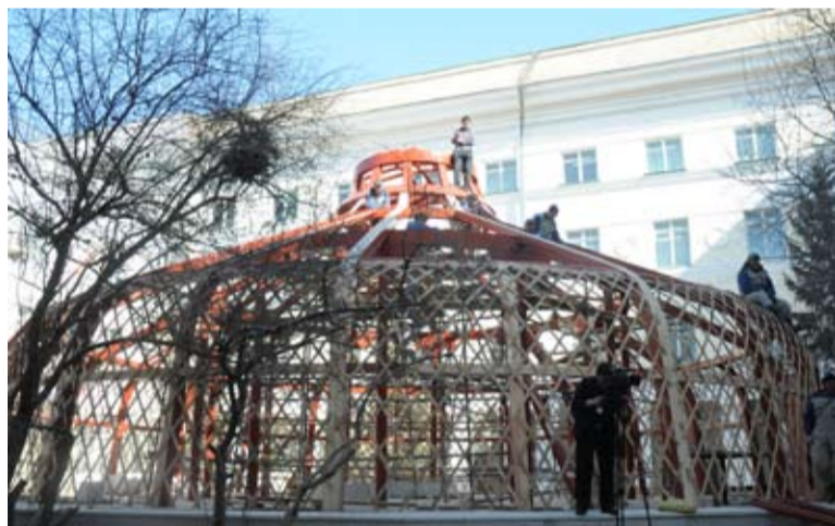
12 Meter diameter gher being erected on State House grounds
